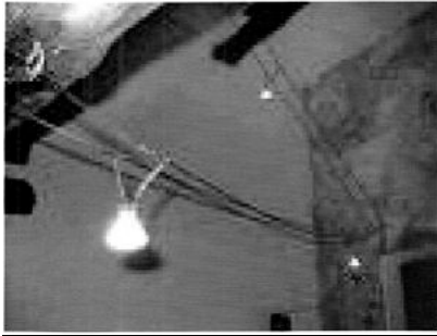
EXPOSED WIRING HAZARD
